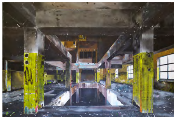
CONCRETE FACTORY - WP20052
